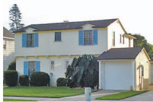
Before the remodel, the Kippurs' 1935 home was closed off to the street. The entrance was at the side of the house. CHRISTIAN RICE
